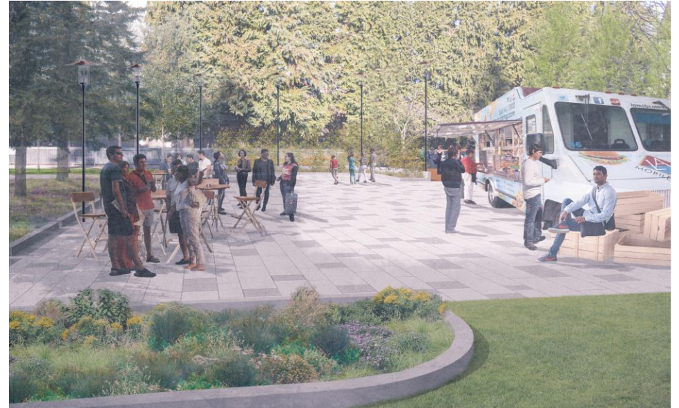
GSI retrofit project that also leverages infrastructure investment with match to deliver on community's 'whole project' vision
