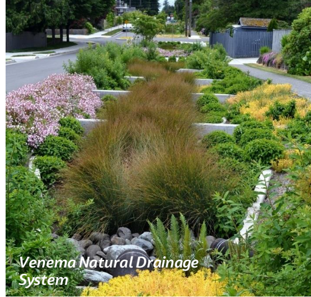
Flow Control/WQ Treatment in the ROW
