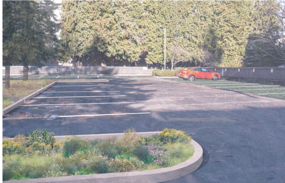
GSI retrofit project that manages runoff to required flow control design standard
