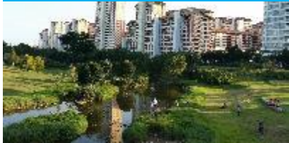
Bishan-AMK Park: integrated with park re- development and drainage- cum-ABC Waters
